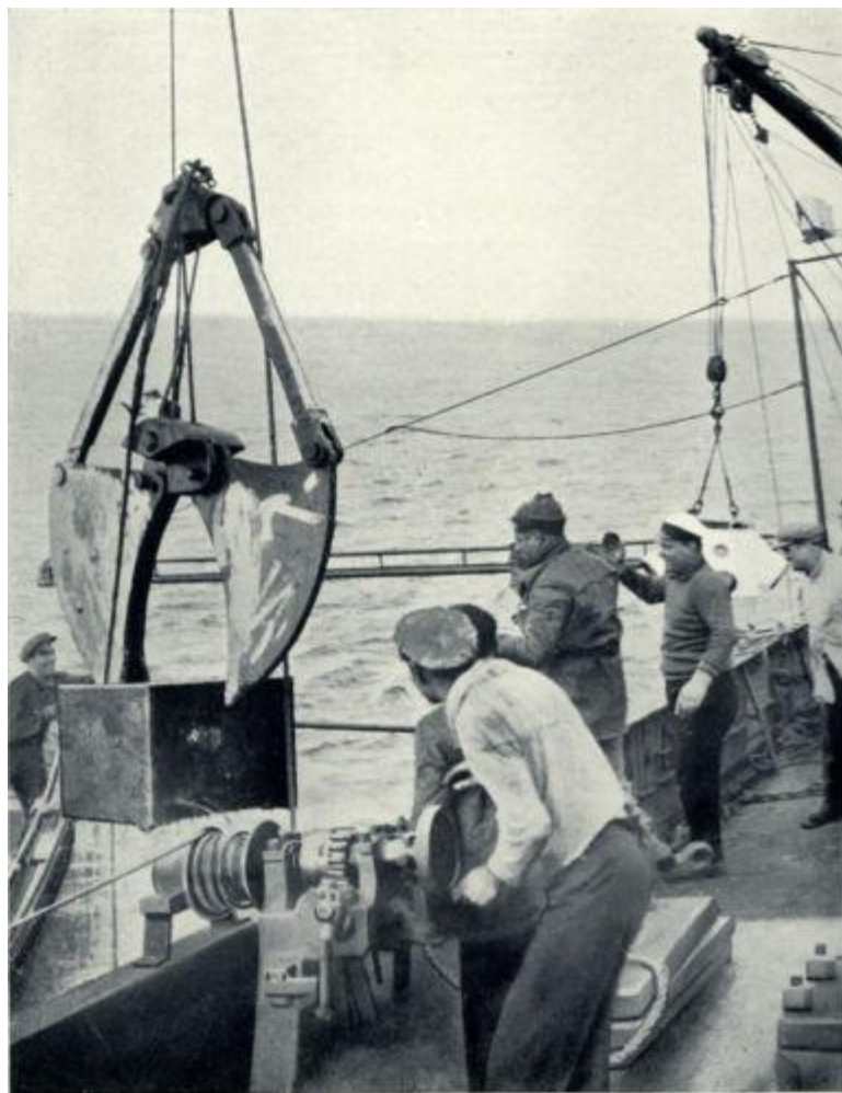
THE CAPTAIN'S SAFE FROM THE 'EGYPT' COMING ABOARD THE 'ARTIGLIO'. NOTE HOW NEATLY THE GRAB IS HOLDING IT
