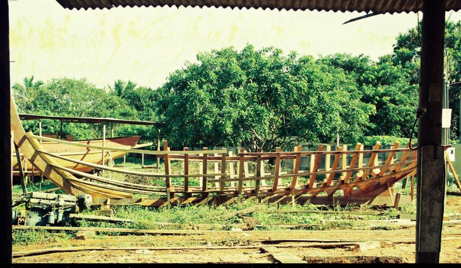
Building with master frames, gauges, and ribbands requires a certain period of apprenticeship to understand the use of geometric aids, which can be used without a full understanding of the geometric steps needed to design the molds, calculate the gauges, or determine the number of pre-designed frames.
